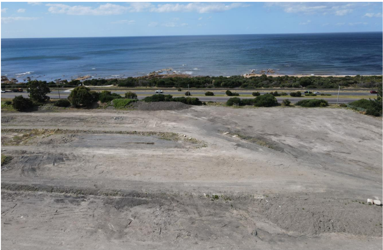
Photo 5-1 Heybridge Converter Station site (where HDD launch pad site would be located), looking north towards Bass Strait
