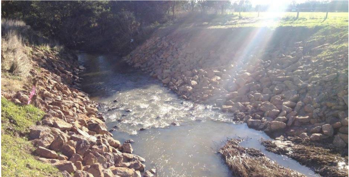
Figure 130. Example grade control structure (rock chute)
