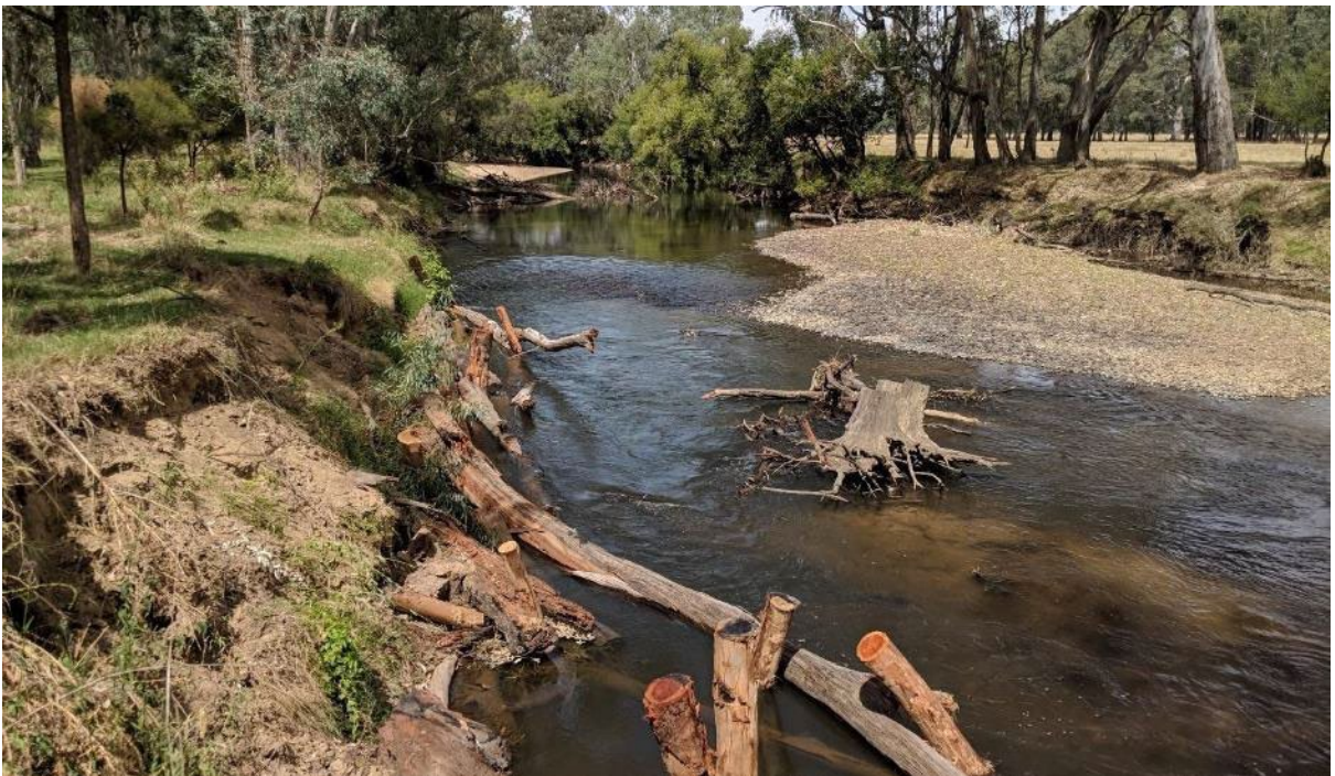
Figure 129. Example of realigned timber to provide bank protection
