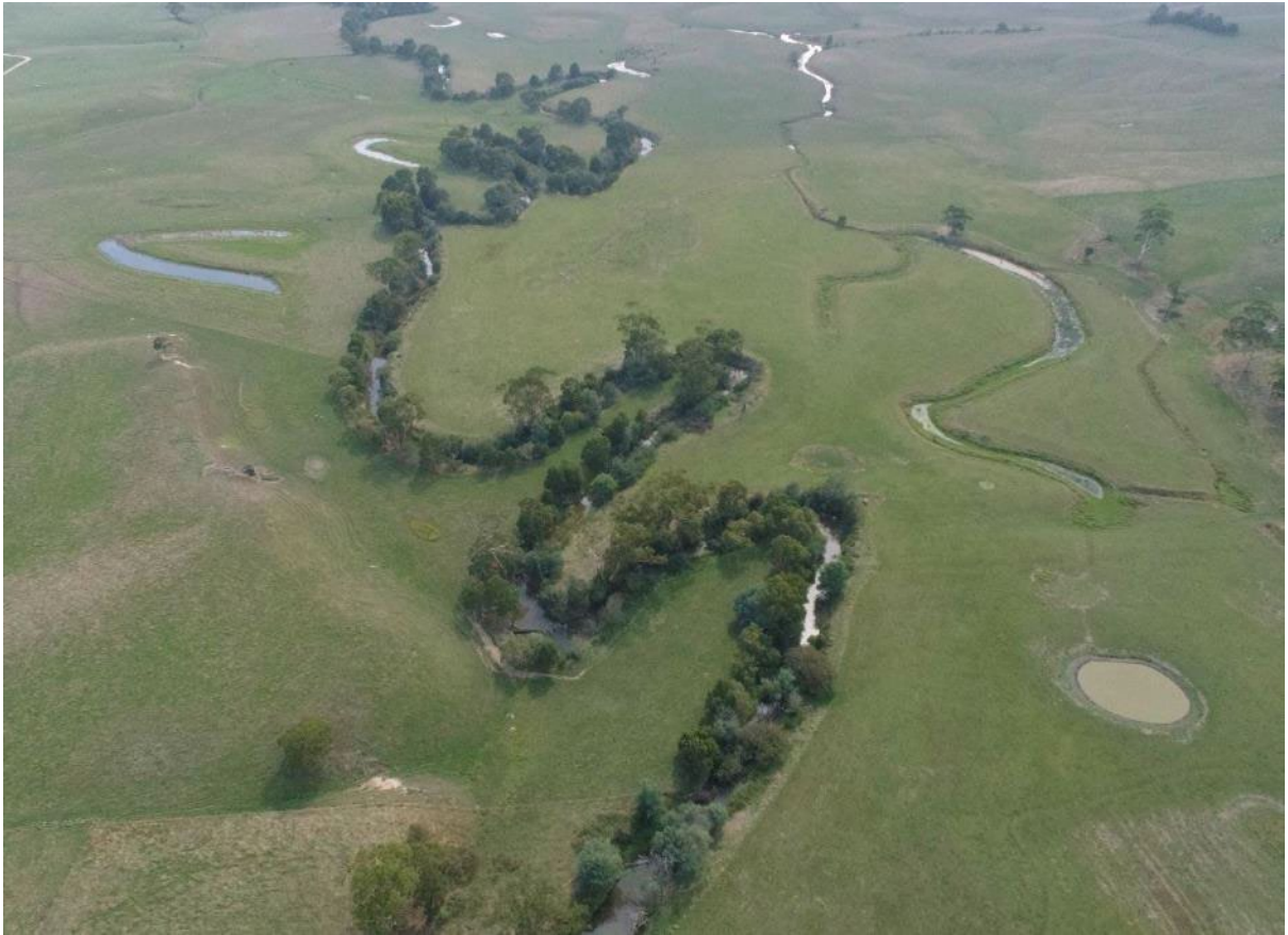
Figure 68. Looking downstream along Morwell River in vicinity of proposed project alignment (fence line near bottom of image)
